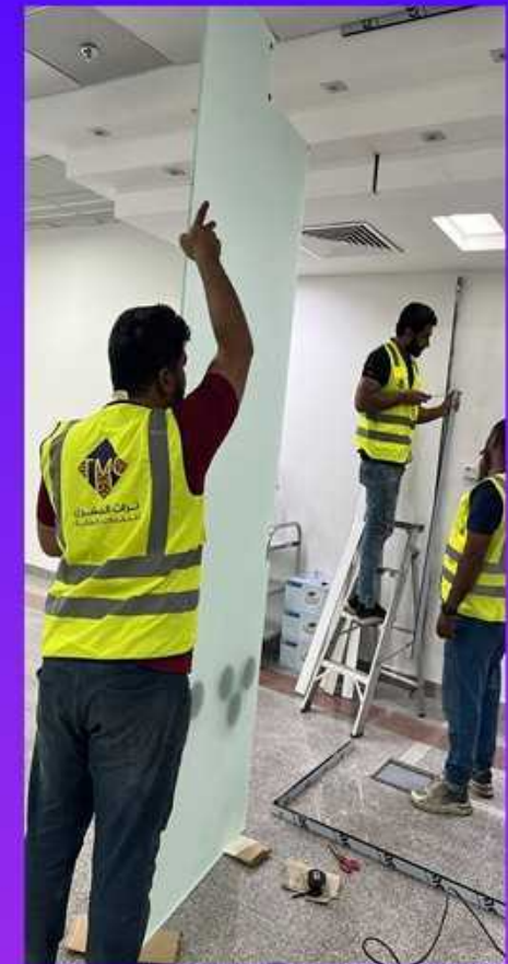
(Ministry of Finance ) Supply and installation of glass partitions in the ministry buildings at exit phase two
