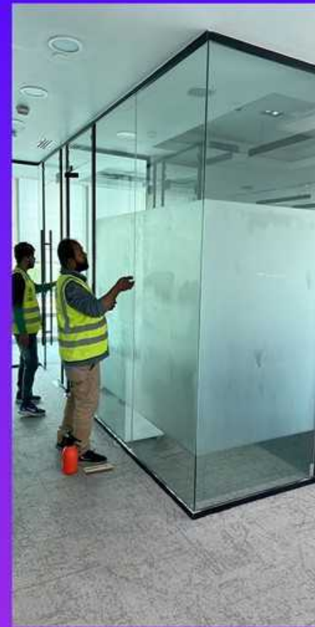
(Ministry of Finance ) Project for the supply ,and installation of canopies aesthetic coverings, and replacement of Lexan panels and sandwich panels in the ministry buildings at Exit in riyadh
